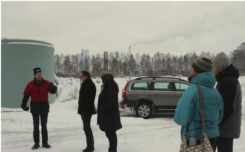
Figure 17: Waste water treatment plant in Enköping
