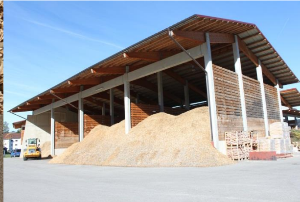
Figure 52: Ideal woodchip storage facility at the Biomass Trade Centre Achenal, Germany (Source: Rutz D.).
