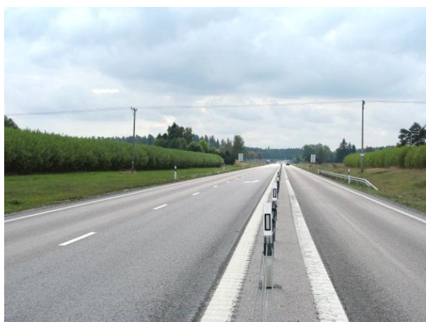
Figure 8: SRC fields close to a bigger road. Wider edges should allow drivers with open views. (Source: Nordh N-E.)
