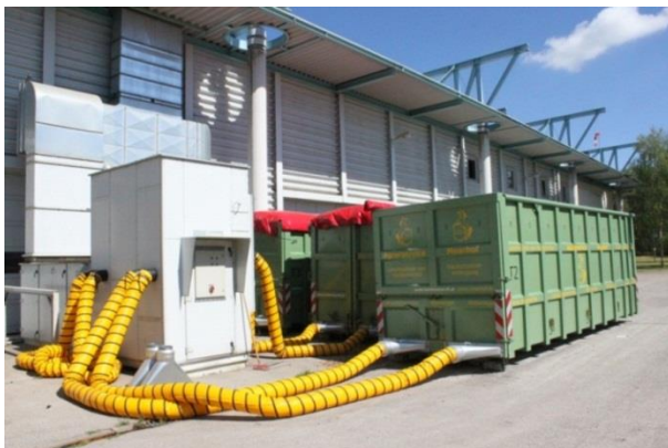
Figure 47: Container and air heating pipes for woodchips drying at a biogas plant in Munich, Germany (Source: Rutz D.).
