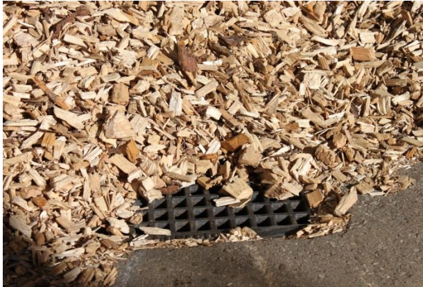
Figure 51: Floor-integrated ventilation slot in the floor of the storage facility of the Biomass Trade Centre Achenal, Germany (see Figure 52) (Source: Rutz D.).
