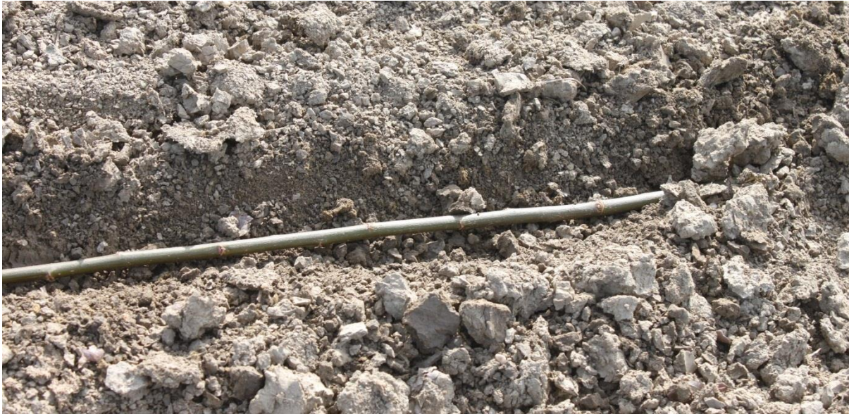
Figure 34: Horizontally laid willow rod: the rod still needs to be covered with soil (Source: Rutz D.)
