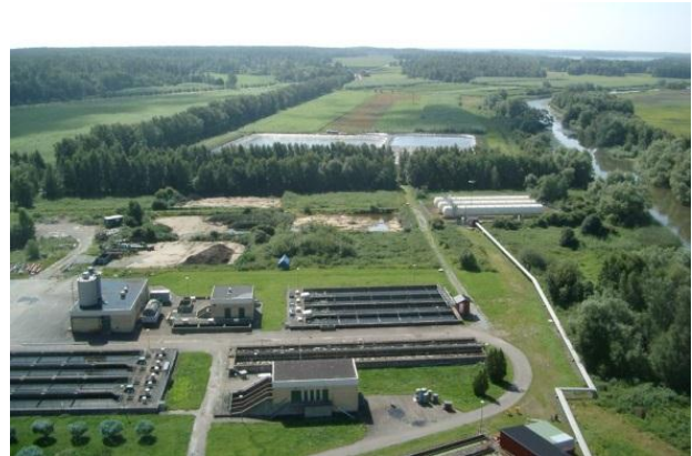
Figure 20: A willow field in central Sweden (background) irrigated with wastewater from a local treatment plant (Photo: Pär Aronsson)
