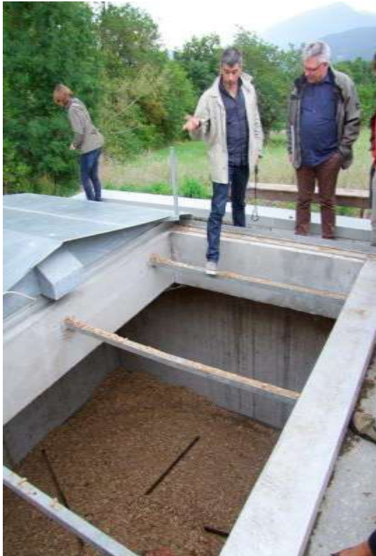
Picture 6: Visiting a wood chip heating system (heating municipal buildings, the library and 3 council flats) in Le Percy
