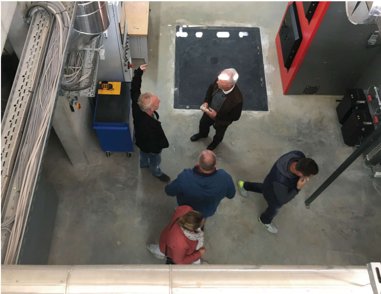
Figure 4: Josef Huber (BAT) explains interested attendants the heating plant, focussing on effects of different wood chip qualities
